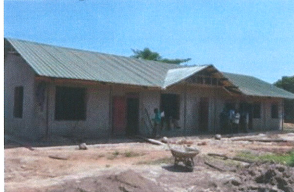
Mukongoro PEAS High School: three-classroom block under construction
