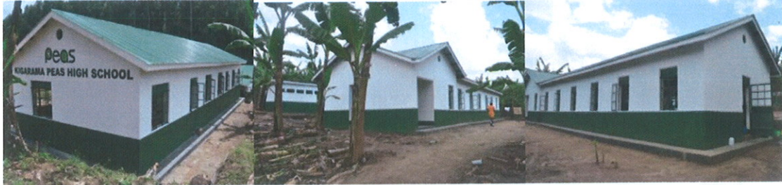
Kigarama PEAS High School: administration block; girl's dormitory; classroom block
