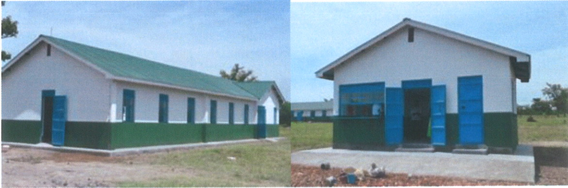
Akoromit PEAS High School: dormitory; administration block
